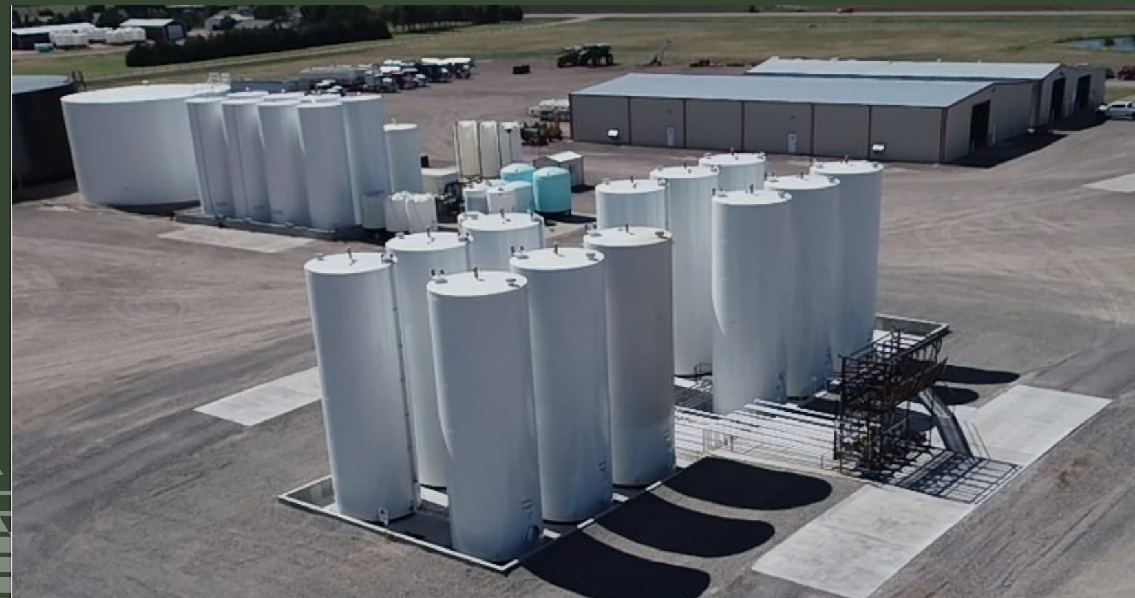
Grant, NE - Bulk fuel plant offering 360,000 gallons of fuel and 60,000 gallons of propane storage.
