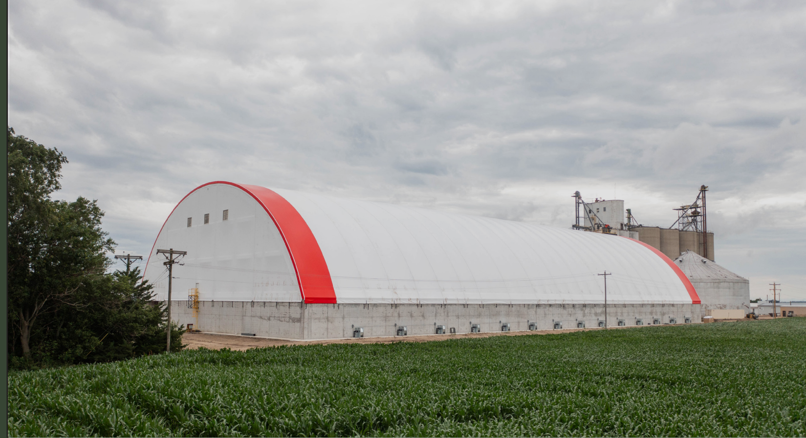
Murphy, NE - 2 million-bushel grain facility, 30,000 bushel per hour leg and outbound scale.
